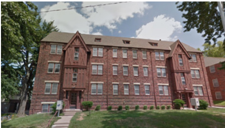
17. Apartment Building (UMM*) 4918 Capitol Ave.
