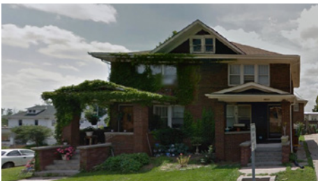
9. Duplex Side-by-Side 4801 Chicago St.
